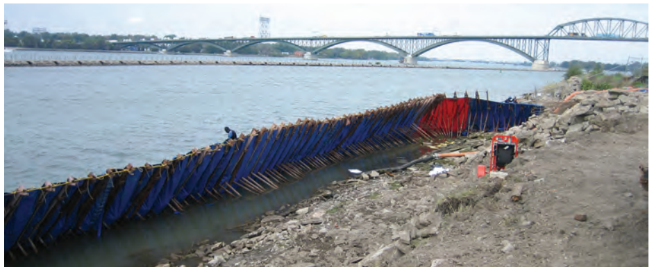
Boathouse under construction with portable cofferdam
