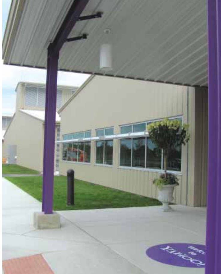
Yahoo’s main entrance welcomes its technical staff and corporate visitors with the impressive visual impact of repetitive structures. Nearly three thousand linear feet of louver banks stretch across the upper and lower levels of the server buildings to facilitate air flow for cooling.
