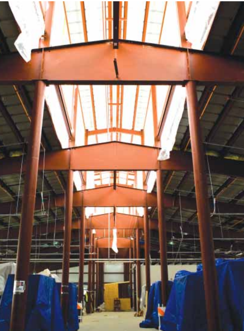
Construction of the "hot aisle" into a contained central area allows heat waste to be ventilated through the cupola louvers high above the server floor, giving the Yahoo Data Center its distinctive "chicken coop" look.
