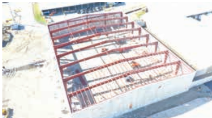
Structural Steel Shell.
