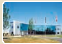
Fujisawa administration building 500,000 man-hours without a lost-time injury
