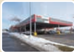
Gordon Food Service Building Conversion
