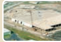
New Plant for McGard First job for Cooper Turbocompressor
